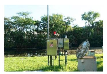
Lift Stations 122, 128, and 210 are being rehabilitated as a part of the City of Sunrise's ongoing sewer collection system rehabilitation and replacement efforts. The City is converting all stations in need of rehabilitation from dry-pit/wet well to submersible in an effort to standardize and improve operation.
